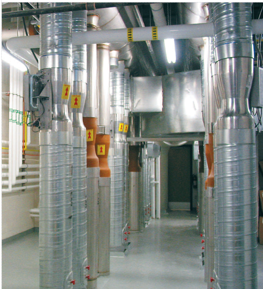
Tracking pairs of patient room venturi valves, which are used for room-level, pandemic-ready HVAC systems.
